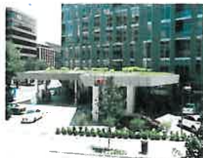
A novel approach was taken to make an Exxon gas station "disappear" from a prime corner site in Washington, D.C.'s West End neighborhood. An irregular bow-tie shaped roof canopy landscaped with a variety of grasses, flowers, and shrubs provides a green visual amenity for occupants of the residential building.
